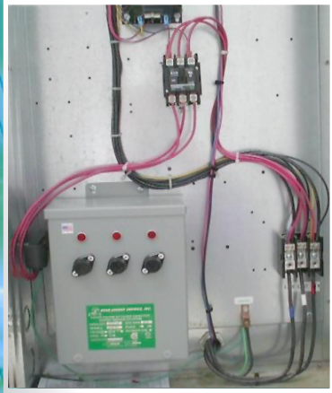
Installed KEC™ Unit
