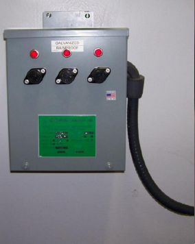
Installed KEC™ Unit
