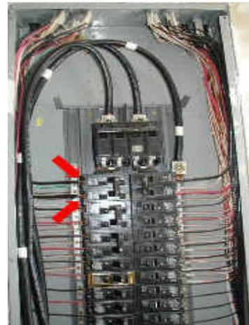
KVAR Energy Savings, Inc. recommends the removal of electrical power to the breaker panel box prior to beginning installation. This is best accomplished by opening the MAIN electrical breaker.
